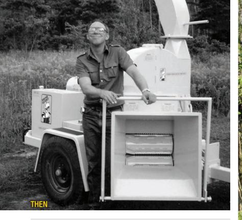
The year was 1983. The very first Bandit<sup>®</sup> chipper was built in a 6,000 square-foot converted repair shop, with the assistance of just six employees. That first machine was the Model 100 Brush Bandit<sup>TM</sup>–a 12-inch capacity, hand-fed disc style chipper (shown here).
